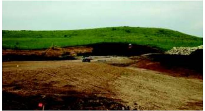
Applying 6"-8" of top soil on the slope behind the stone retaining wall of the parking lot, June 13, 2018.
